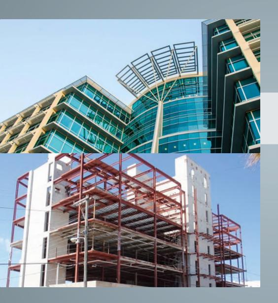
Above Left: Finished Facade Below Left: During construction, showing the concrete elevator cores and light steel frame designed by
